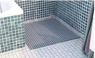
Example of a typical shower unit. A shower tray like this one will be filled up with tiles and if necessary fitted with a small ramp if necessary.
